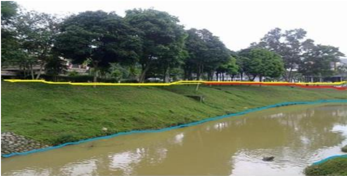
Figure 3. Corridor zone in UTM River
